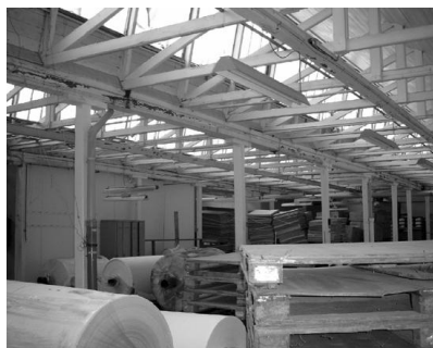
Fig. 4 Grenaa Textile factory the inside of the factory.
