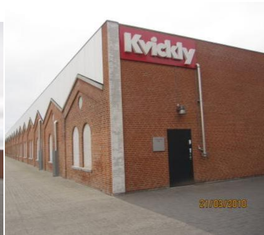
Fig 11. The new supermarket with the gables of the former building attached
