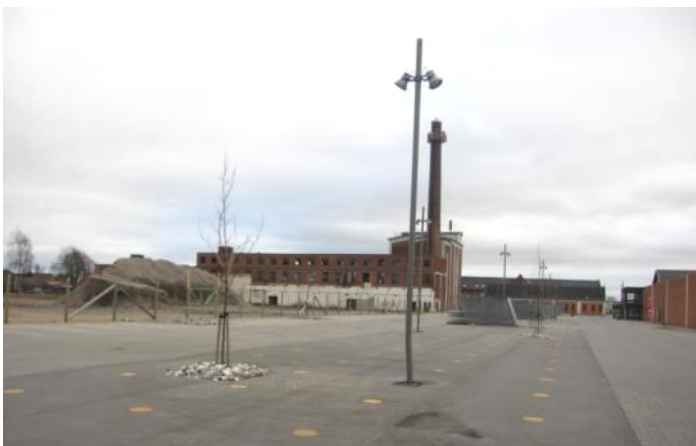
Fig 10. The site today, most of the building has been removed.
